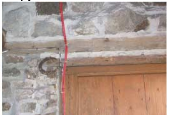
View of north plate from inside shed. Plate stops well before brick flue of beehive oven to left. Door to room “B108” is positioned just below plate.
