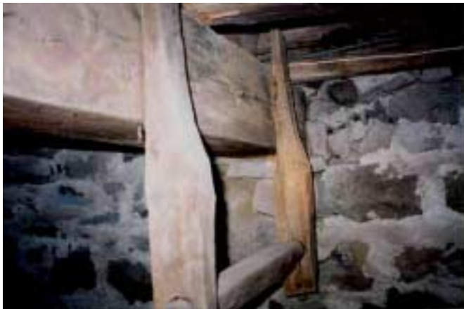
Storage rack hanging from central East-West summer beam under 1st floor joists in "B0" cellar. West end of beam rests in large pocket on west wall. (Other end is embedded in fireplace mass.)
