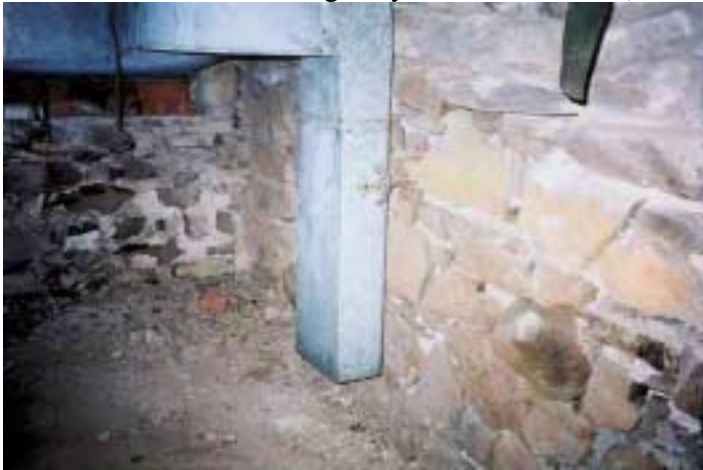
North wall & crawl-space entrance visible under duct work. Vertical duct abuts west face of "B0" fireplace mound hearth extension. Note variation in hearth extension finish.
