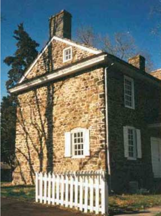
West end unit "A". Note Garret SW window, protruding ledge cornice. Once the east end of unit "A" looked like this, rotated 180° – it had a NE garret window. Note darker chimney stone.
