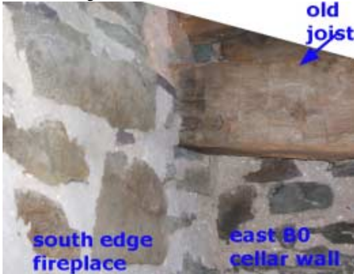
Close-up of old floor joist along east wall of "B0" embedded in south end of fireplace mass. Current floor joist directly above it.
