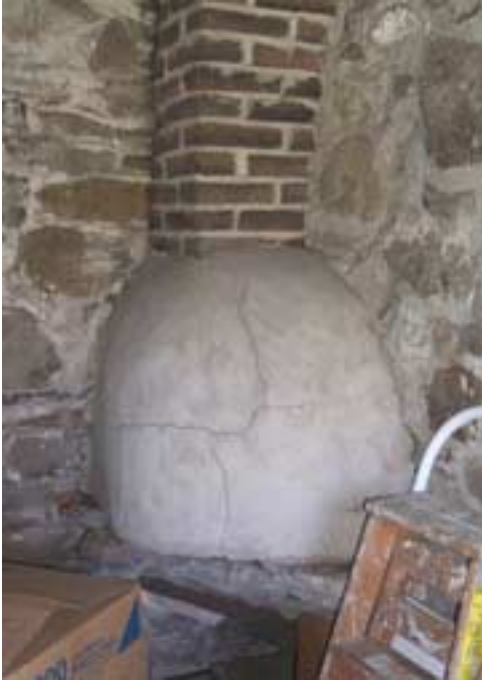
Exterior and brick flue of beehive oven
