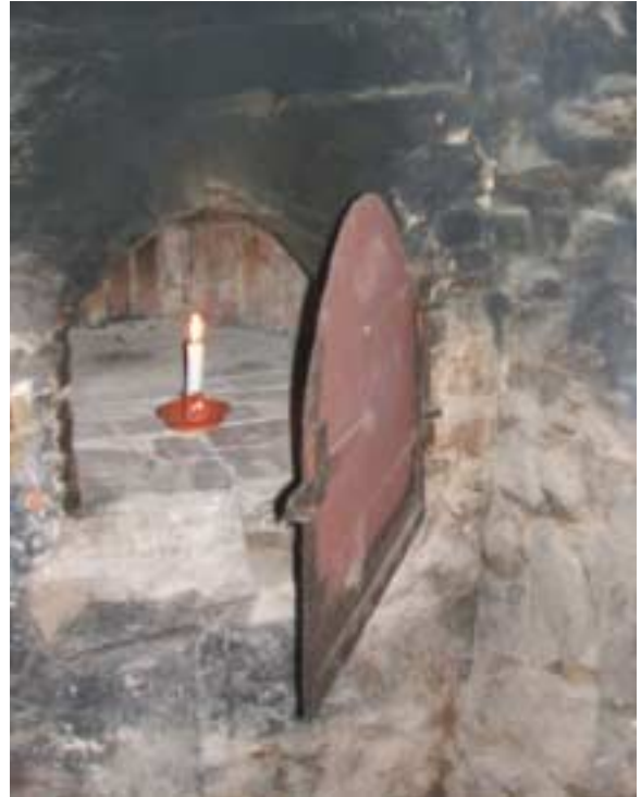
Beehive oven in north jamb of "B1" fireplace
