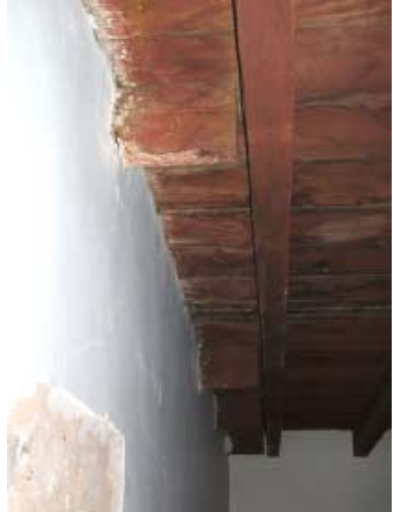
Unit "B", 2 nd floor shows East cornice supports protruding from the west wall, which once was the exterior wall of unit "A". The cornice protrusions are not supporting or connected to the unit "B" garret floor joists, that make up the ceiling.
