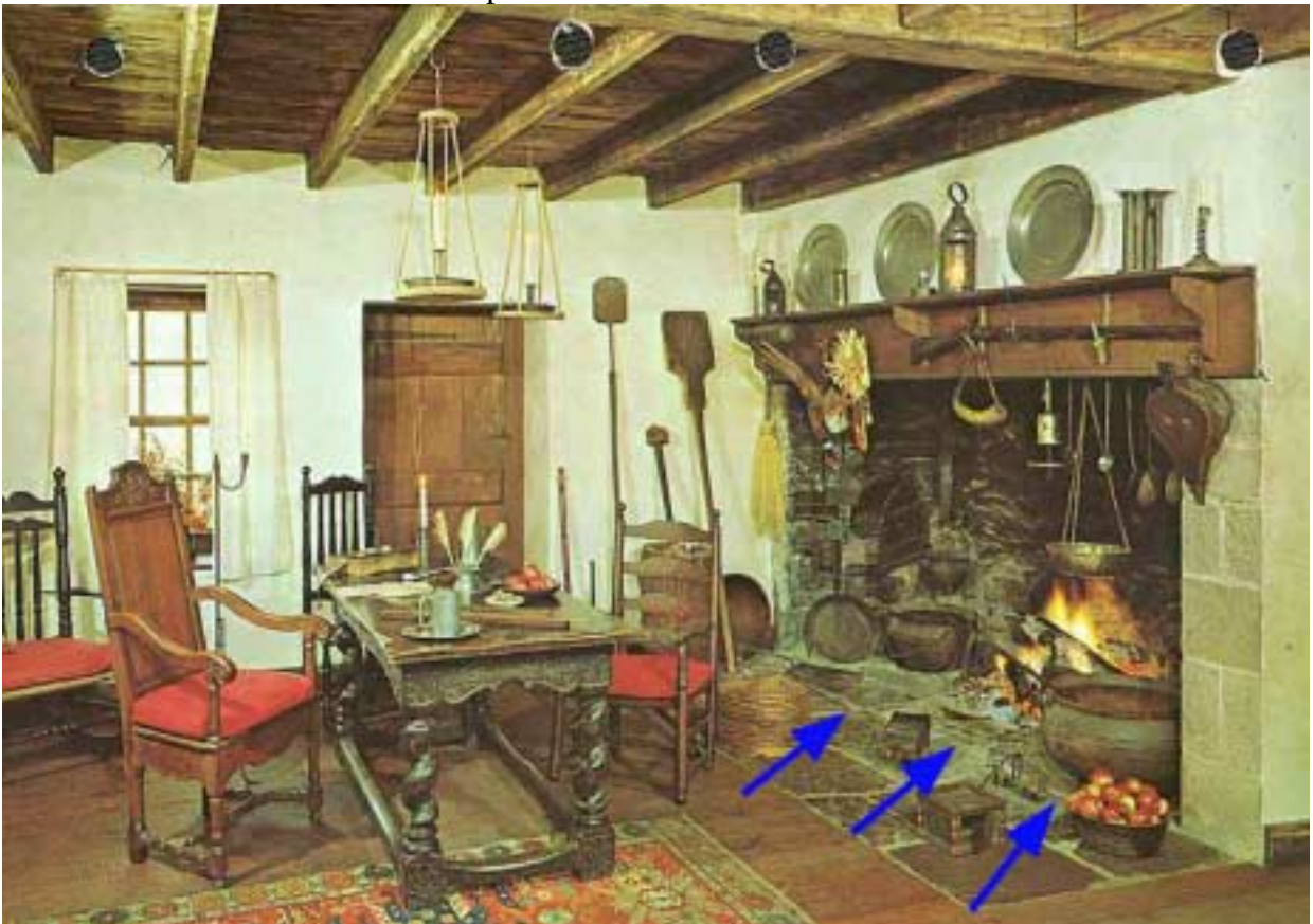
Blue arrows highlight north-south seam in hearth indicating area extending into the room is an addition.
