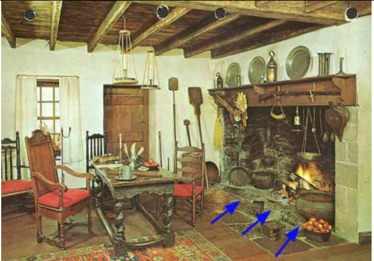
Blue arrows highlight north-south seam in hearth indicating area extending into the room is an addition.
